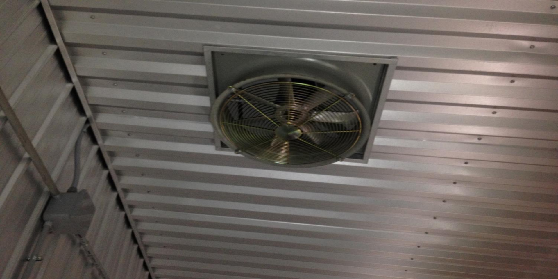
Air wall with computer controlled fan for condensation management
